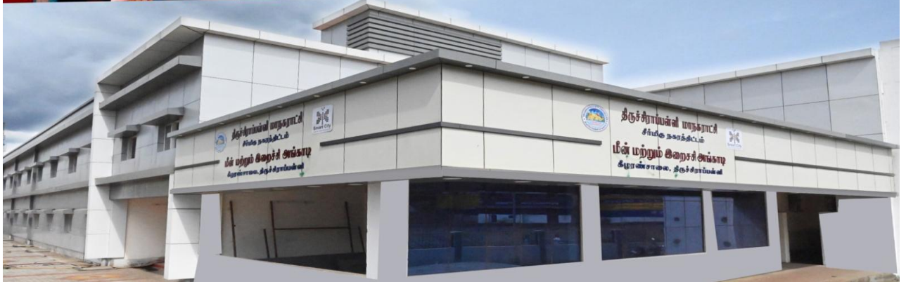
Fish and Market Market constructed under Smart City Mission was inaugurated
